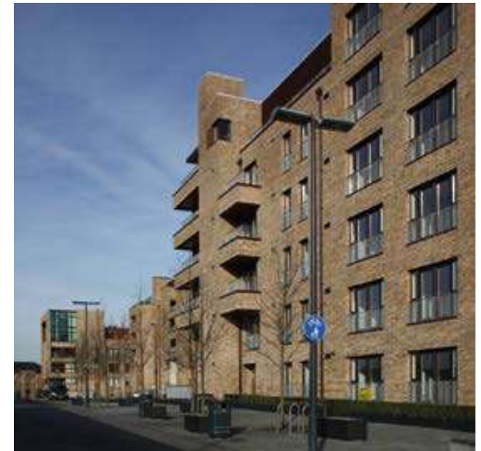
Modern use of brick in an historic environment—McEwan Square / Fountainbridge Brick has been used to integrate this development into its historic surroundings. The development is overtly contemporary in its appearance. The colour of bricks was chosen to harmonise with the stone of the adjacent tenements. Combined with the vertical emphasis to the window and the building's scale, the material choice has helped ensure this development adds to Edinburgh's sense of place. This development sets the standard for the use of brick within Edinburgh.
