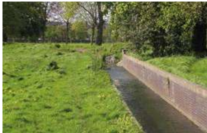
Inch Park Removal of a straightened and modified channel along the Braid Burn at Inch Park and re-meandering to create a natural watercourse with riffles, pools and vegetation as part of flood prevention works.
