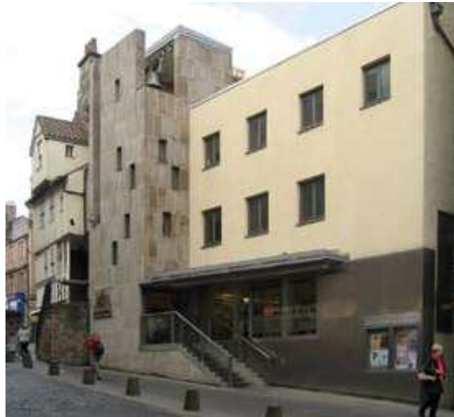
Integrating the new with the old - High Street
