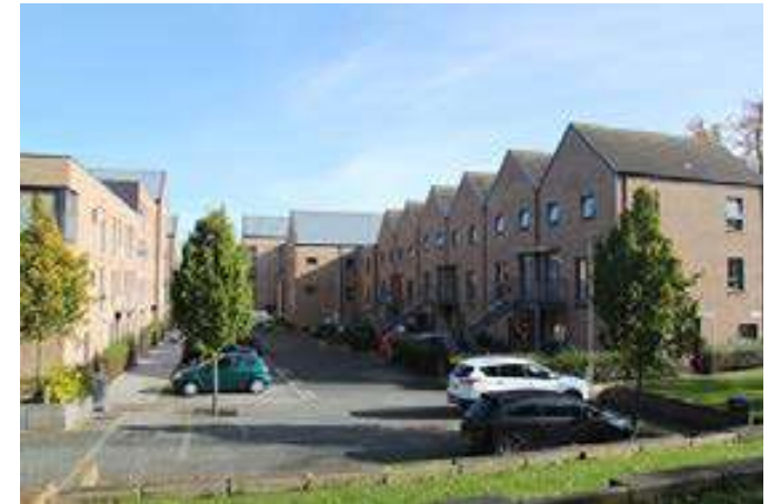
Minimising energy use through careful design—Garvald Street This housing development achieved a BREEAM excellence award in recognition of its high standards of sustainability. It achieves this through a range of measures including insulation, airtightness and heat recovery.
