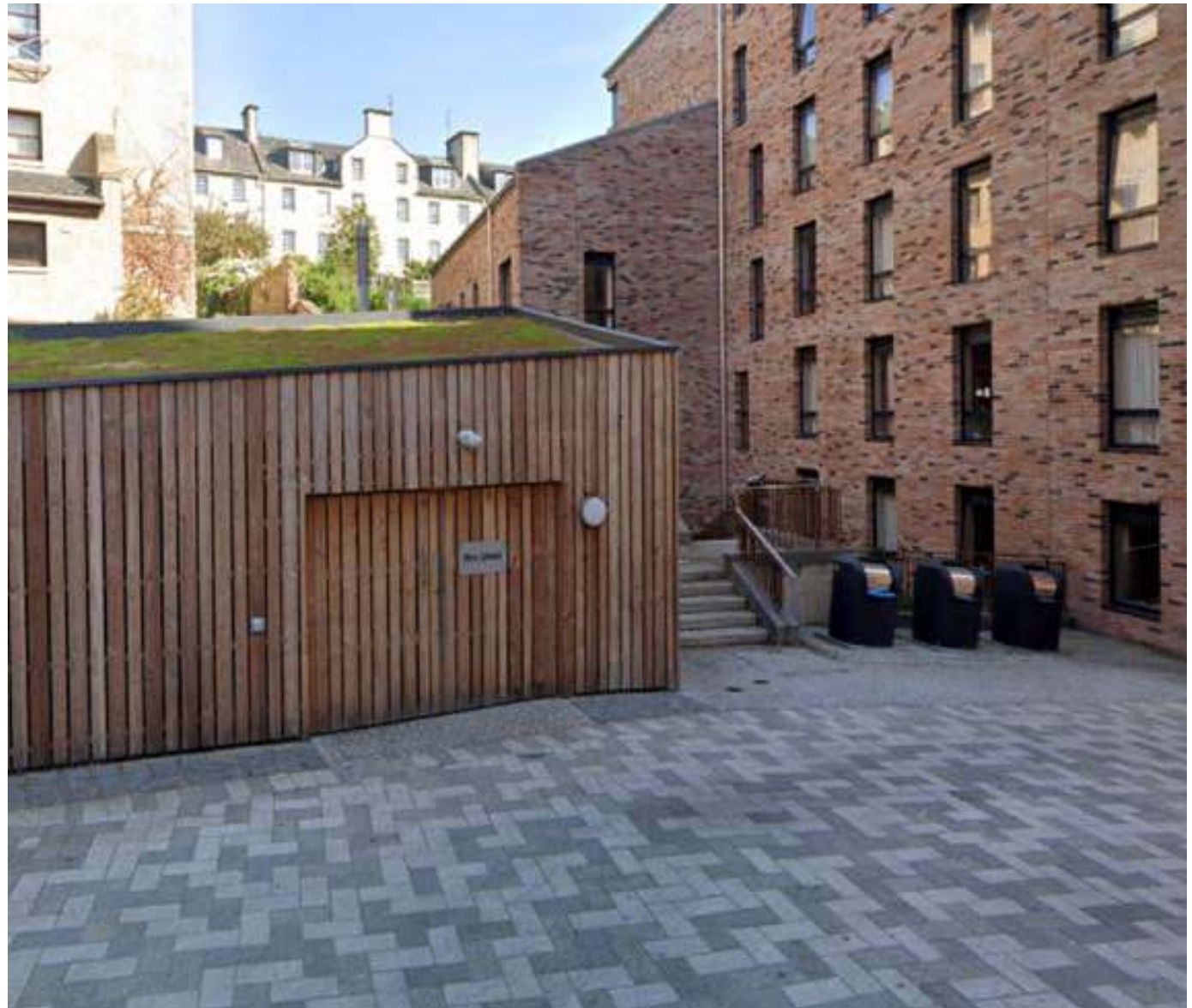
The use of bins with underground storage at Morgans Lane helps to minimise the impact of waste collection facilities.
