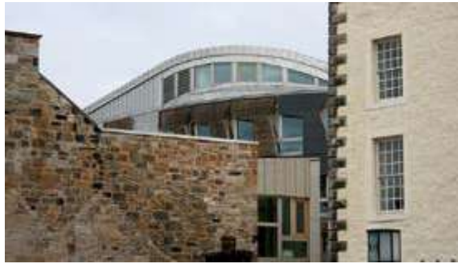
Metal roofing in a historic context — Canongate Stainless Steel roofing has been used on the Scottish Parliament.
