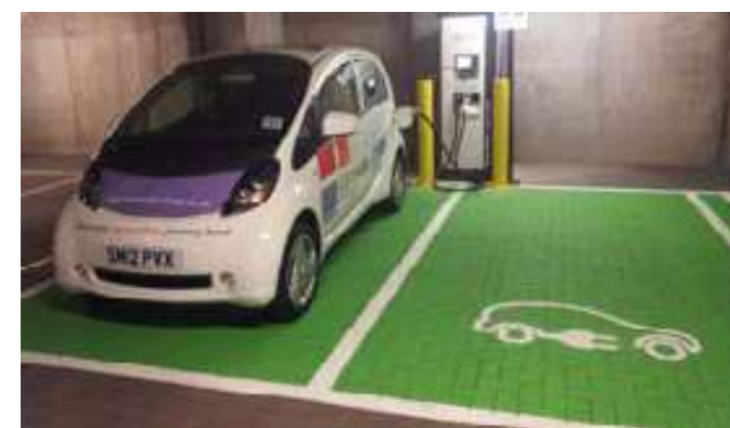
Fountain Park installation of underground car-park electric vehicle charging.
