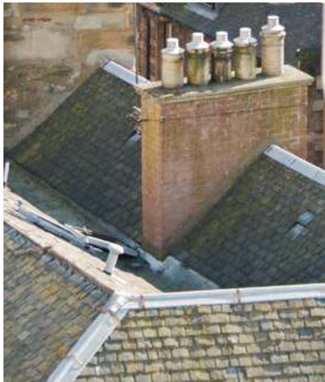
Traditional roofing materials Slate, Lead and zinc are traditional roofing materials used in Edinburgh—seen here from the Museum of Scotland's roof.
