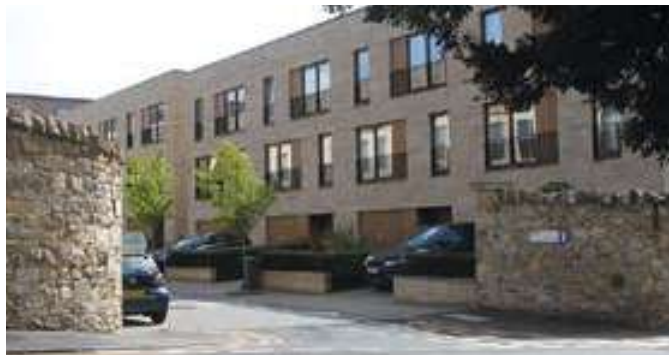
Strong boundary treatment and landscaping define plots and reduce the visual impact of parked cars at Wallace Gardens
