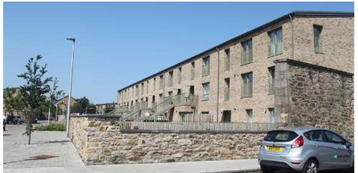
Incorporating existing features and boundary walls—Leith Fort Existing lodge buildings and perimeter walls preserve the heritage of the area and give character to a new housing development.
