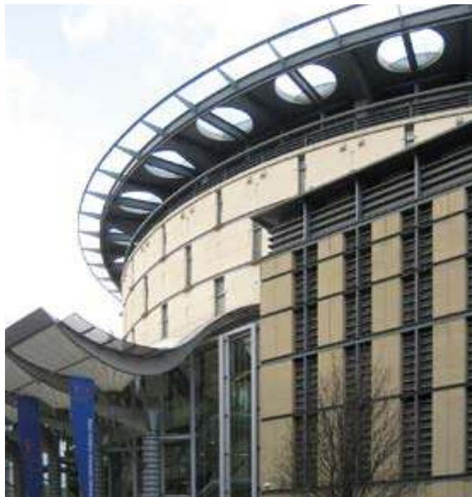
A mixture of cast stone & natural stone—Morrison St. Cast stone was used at high level on the drum shaped part of the building while natural stone was used at low level on the corners.
