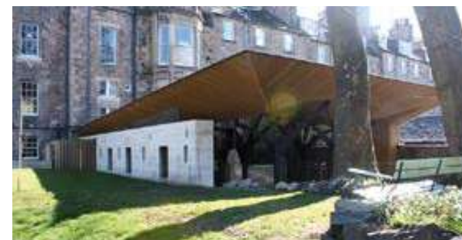
Frameless glazing - George Square Lane Glazing is used to create the effect of a floating roof on this building.
