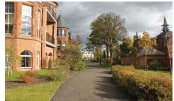
Former City Hospital - Greenbank
