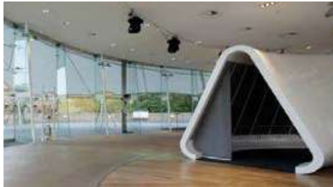
Good design for noise was used at Our Dynamic Earth to stop noise escaping from one of their function areas. Instead of installing doors they installed a triangle, zigzagged corridor.
