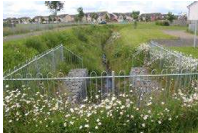
SuDS retention basin and swales, Kirkliston
