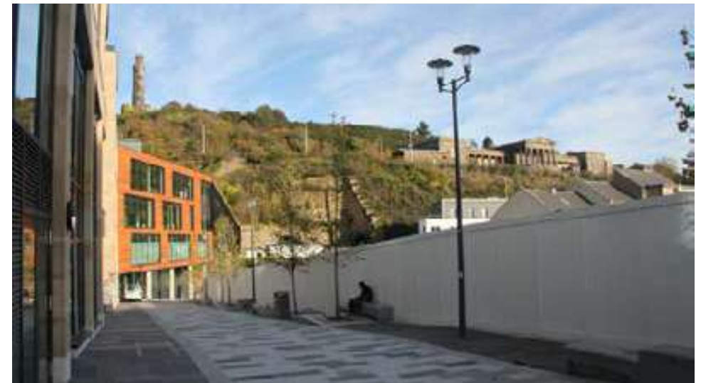
New public realm and link created between Canongate and Calton Road (the building on the right is still under construction).
