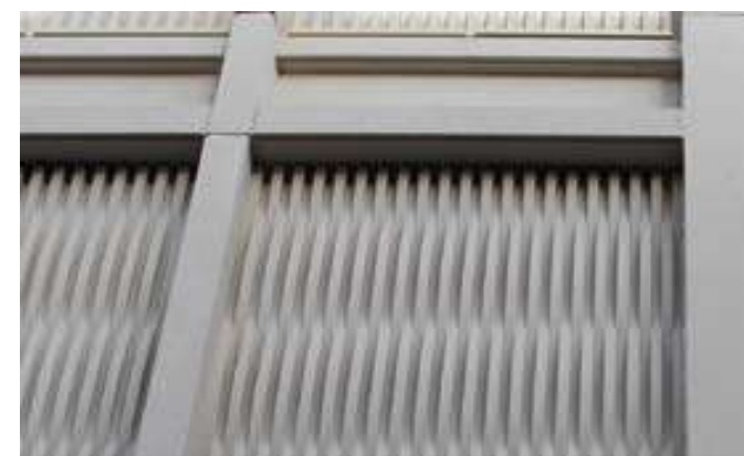
Textures created with concrete—Princes Street Concrete panels with a textured surface treatment are used on this recent building on Princes Street.
