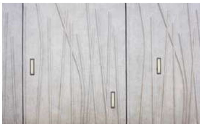
Concrete used sculpturally—Horse Wynd The sculptural potential of concrete is exploited in the Parliament wall with the patterned surface and integration of lights
